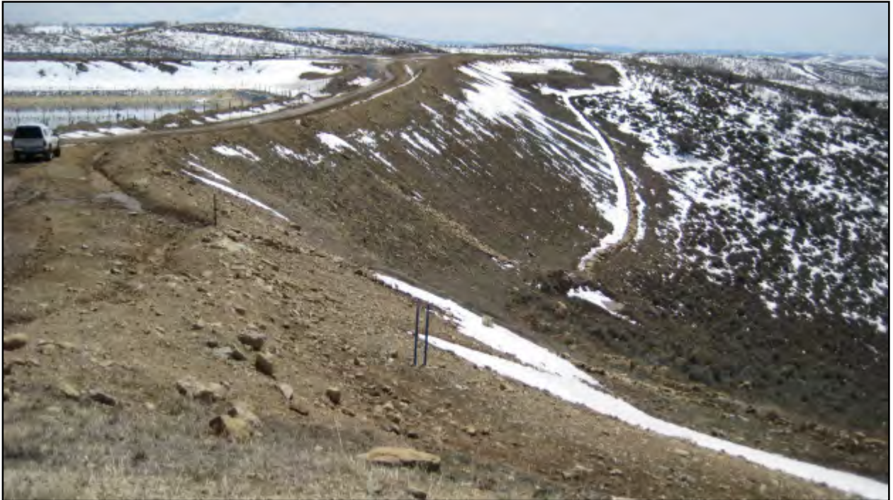
Photo 1. Looking southwest from northwest corner of Oxy Pond 13 project area (4.24.13).
