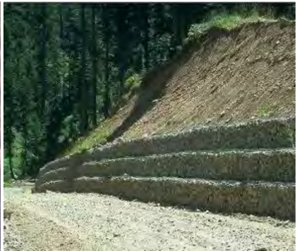
Gabion Retaining Wall
