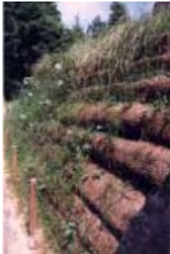
Timber Retaining Wall
