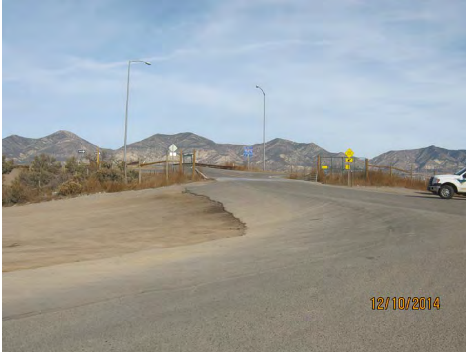
PHOTO 1: West leg looking north onto County Road 315 from County Road 346.
