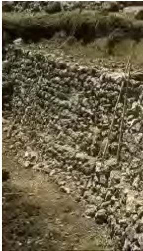
Rock Retaining Wall
