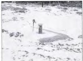
Typical Well Head Photo Showing 4' x 4' Concrete Pad with Watertight Well Cap Casing to be a min of 12\"/>
